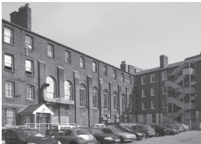
The rear elevation of Block B.
