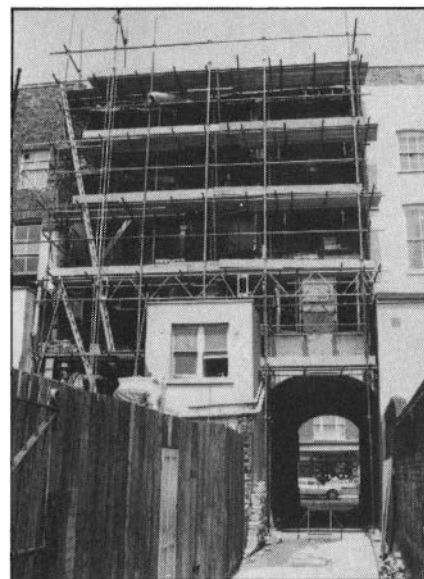
The rear of the house during rebuilding.
