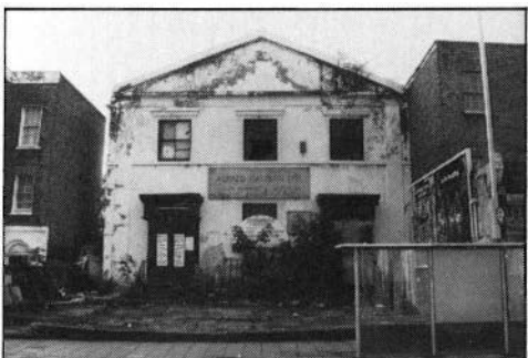
The Non-Conformist Chapel at 47 Balls Pond Road being used as a furniture warehouse.
