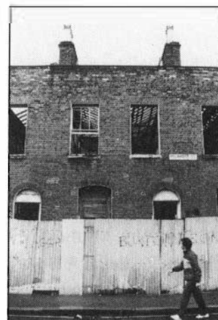
7-8 Micawber Street back from the brink. Renovation is now in progress.
