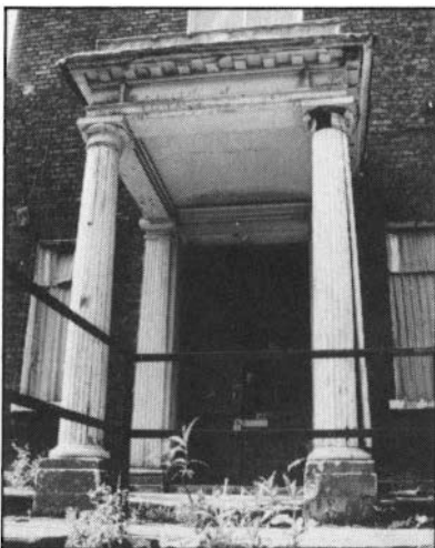
The front of the building prior to collapse during conversion works. The entrance porch is in the Doric style.
