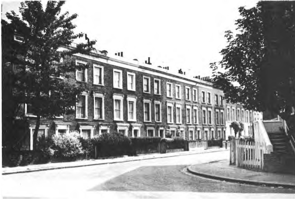
Shakspeare Walk itself showing some of the better houses with their elegant and balanced proportions.
