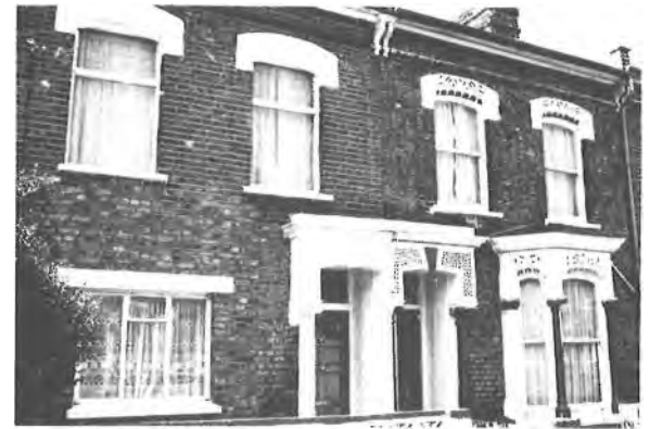
Removal of the bay window flattens the front of the house, reduces the size of the front room and cuts out light.
