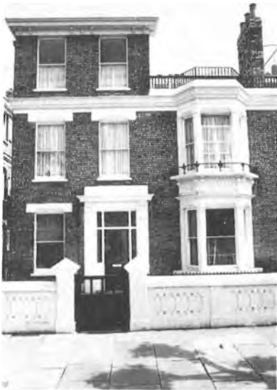
House in Bethune Road showing the grander style of these large Victorian houses. Careful detailing of bands of plasterwork binds the different storey heights together.
