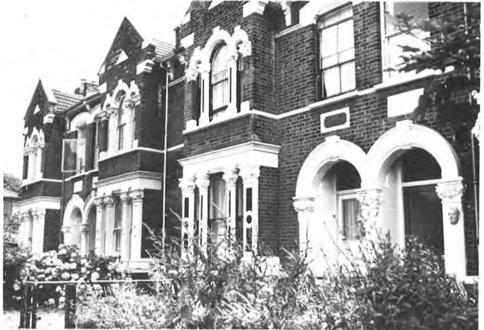
Houses in St. Kildas Road with ornate plaster work details around doors and windows. Each house has small variations in the detail work.
