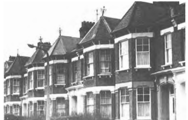
Houses in the same area with simpler rooves and plasterwork arches over doorways.
