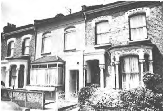
A badly proportioned new window that destroys the balance that existed in the original house.
